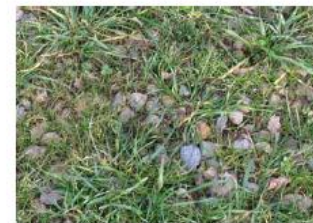
parking terre-pierre enherbé
